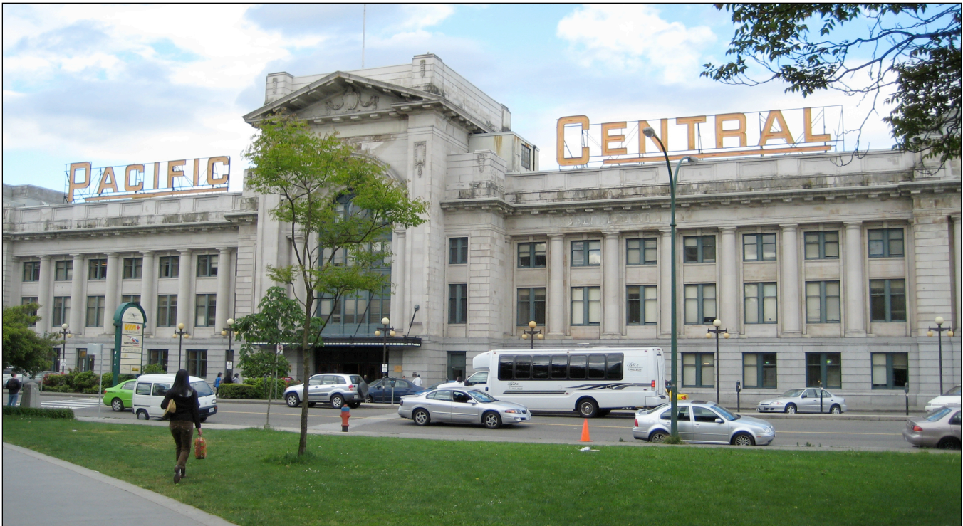
Pacific Central in Vancouver, BC is home to Greyhound, VIA Rail and Amtrak. Why then does the Canadian Border Security Agency consider this a “new” facility for a 2nd Amtrak train? More on Page 6. Photo: Jon Calon
